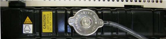
To check the coolant, remove the cap from the top of the radiator (\*) **ONLY when the set is completely cold**, and visually inspect that the coolant in the radiator is visible above the radiator elements. If coolant is required add until the level reaches the base of the filler neck. Replace and tighten coolant cap on top of radiator.
